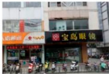
3.1 Extensive windows along the street (ratio of windows in the SVI)
